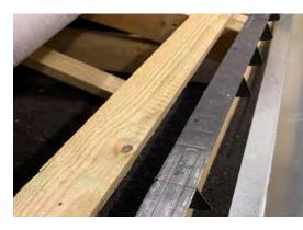
**2** Eave Tray must be set square to the eaves and secured into the eave batten.
