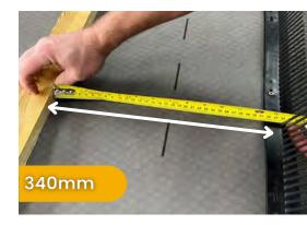
2 Install the next batten with a measurement 350mm up from the bottom of the first batten.
