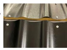
2 The sheets need to be 20-25mm short of the ridgeline and the membrane is 10-15mm short.
