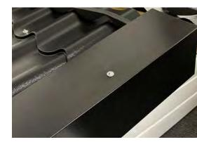
2 For multiple flashing, lap by 100mm. Repeat the process until the flashing exceeds the ridge line.
