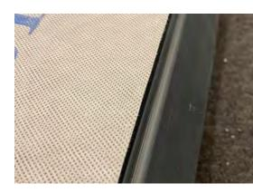
4 Install the comb filler on top of the eave tray in line with the downturn.
