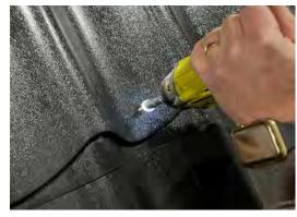
**3** The fixing has a rubber washer, which allows the fixing through the pan.
