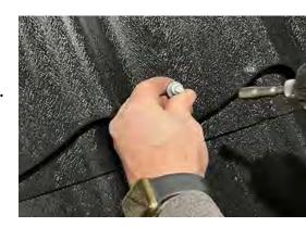
2 Using an 8mm bi-hex head drill bit in an impact driver, secure the fixing.
