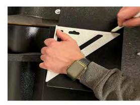
**3** Mark a line on the excess, in line with the ridgeline and vertically down the gable.
