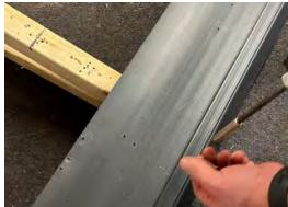
3 Lay the membrane over the eave tray, making sure it's aligned with the downturn of the eave tray.
