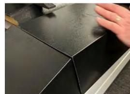
**4** Cut the verge flashing, with tin snips or similar and reposition so that the gable end is covered. Secure as previously stated.
