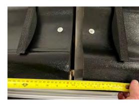
4 Place the ridge flashings with the centre of the flashing in line with the ridge line. Secure with fixings approx. 500mm apart through the crown of the sheet and into the verge flashing.
